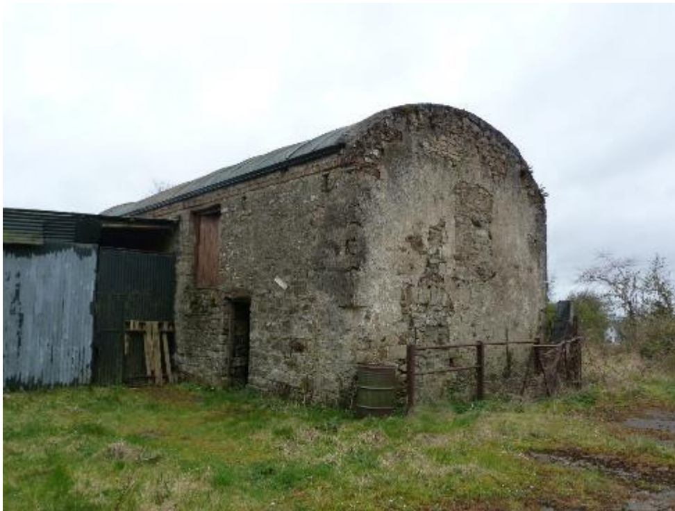
Plate 14-4 Field 5 Castlegal House, outbuilding (AHC 41)
