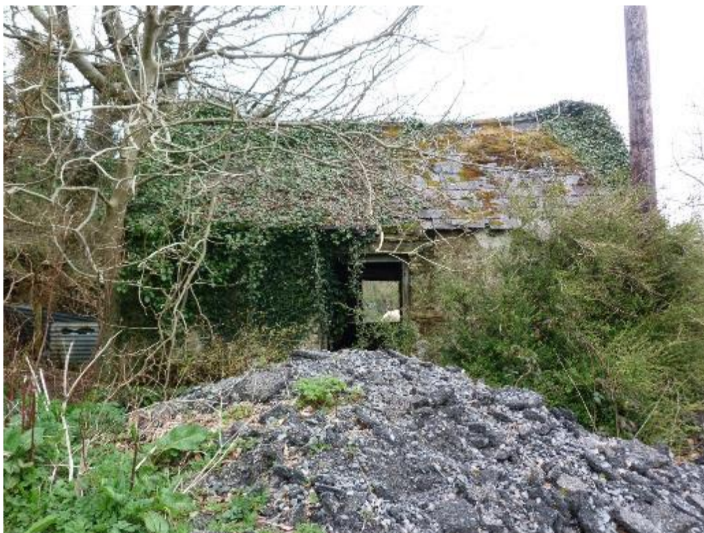
Plate 14-11 Field 11, house (AHC 44) from north
