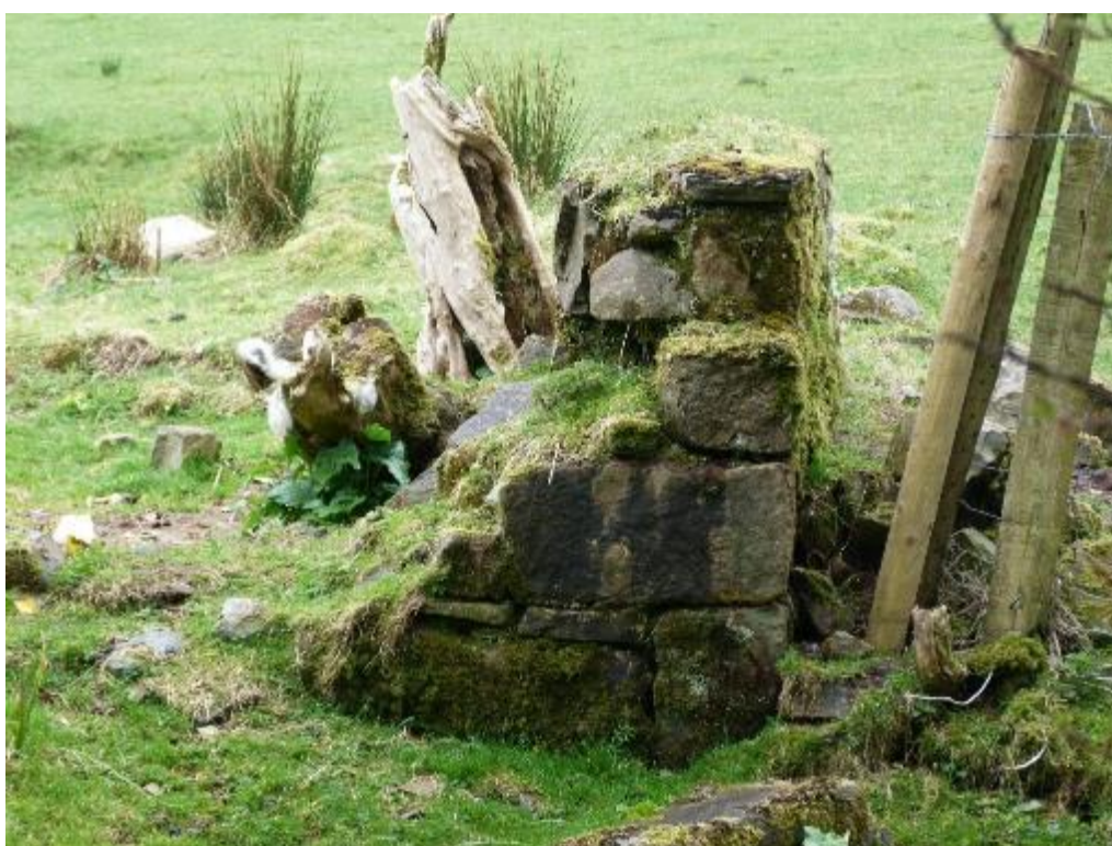
Plate 14-8 Field 10 standing remains of building (AHC 42)
